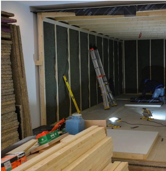
Figure 3 The view of a room-section during construction, showing the sandwich floor, the walls, and the ceiling.
