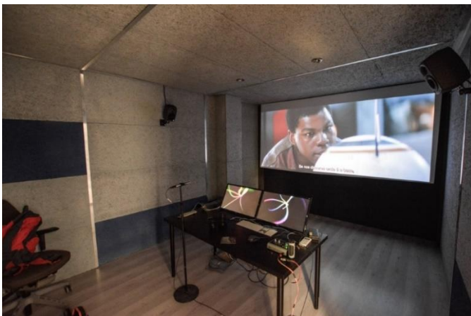
Figure 4 The interior of a finished room in Lisbon, lined with Celenit AB
