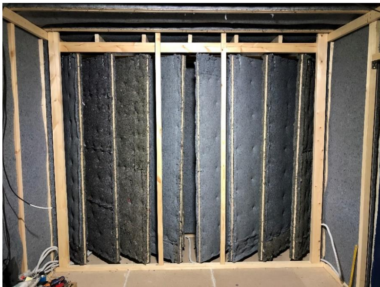
Figure 5 A rear-wall wide-band absorber, as typically used in a control room or a dedicated voice-over room
