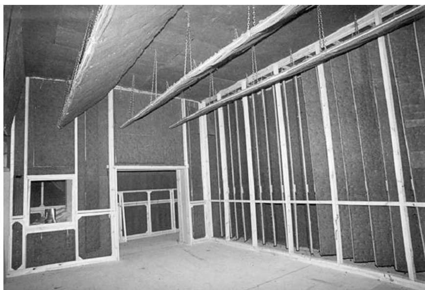
Figure A.1.10: The completed acoustic treatment, viewed from the monitor loudspeaker wall.
