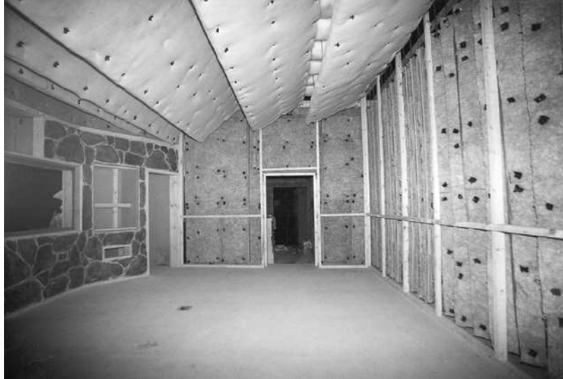
Figure A.1.11: The completed acoustic control system at Area Master Studios (now Planta Sónica 2), Vigo, Spain; viewed from the rear, and showing the closed nature of the ceiling panels from this viewpoint. Compare this with the view in Figure A.1.10.
