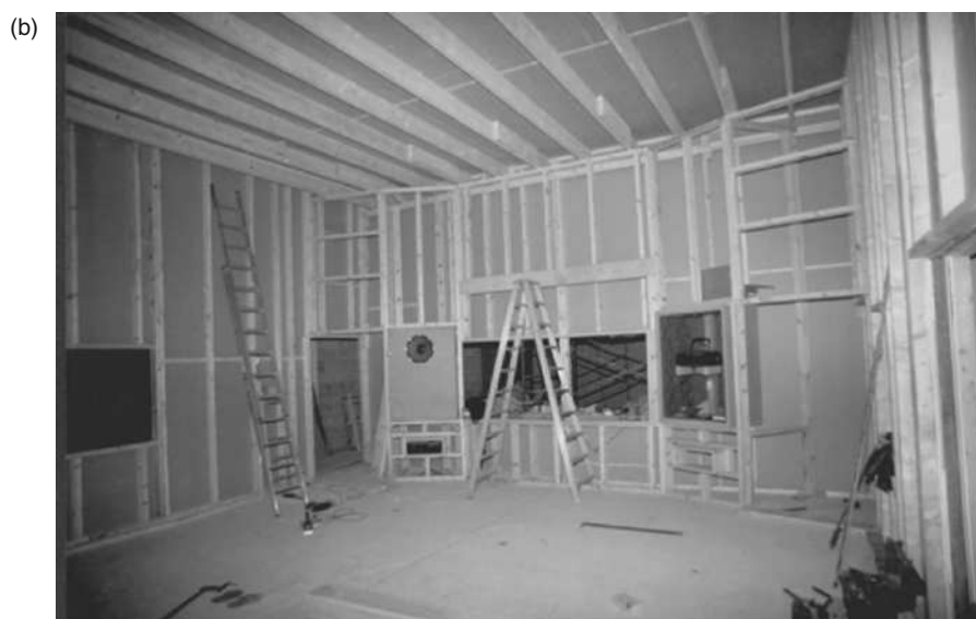
Figure A.1.9 (continued) (b) The loudspeaker wall framing at the stage of Measurement No 3.
