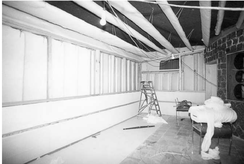
Figure A.1.12: Discosette 3, Lisbon, Portugal; at the stage of mounting the first fabric panels over the absorber systems. The floor is pink marble. The covering on the waveguide panels is Dacron.
